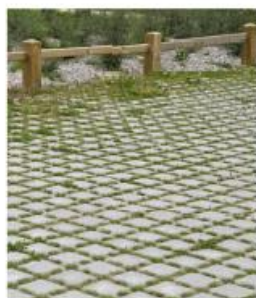
Dalle béton - joint gazon
